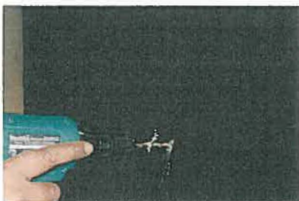
Through panel diagonal lap joint
