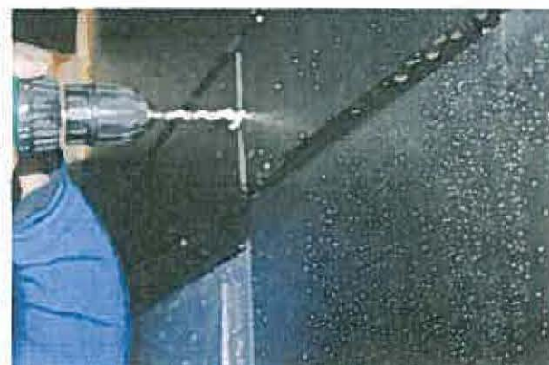
Through panel vertical lap joint
