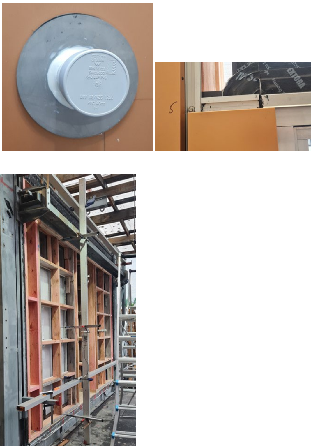
Figure 3: Selected Photos from Testing
