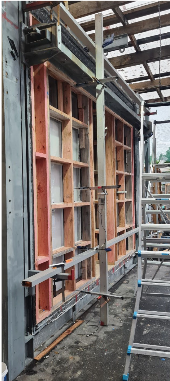
Figure 2: SLS displacement transducers on stud
