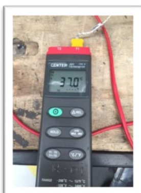
Figure 4: Temperature of outer flue 37.0 °C
